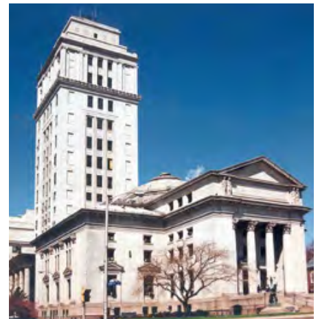
The Union County Courthouse in Elizabeth as it appears today.
